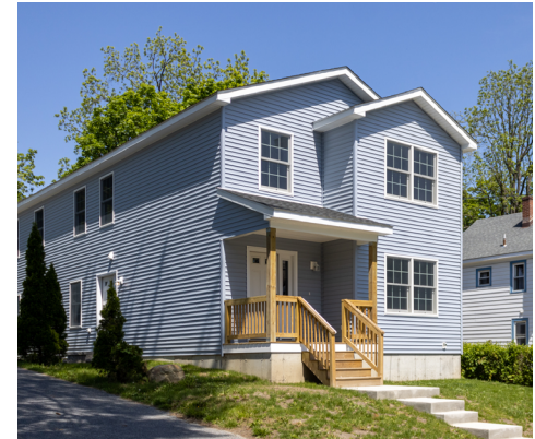
One of three new two-family homes built by Hudson River Housing for first-time homeowners in Poughkeepsie's Northside neighborhood. Prospective buyers will receive homebuyer counseling and landlord training from the NeighborWorks HomeOwnership Center of Dutchess County.
